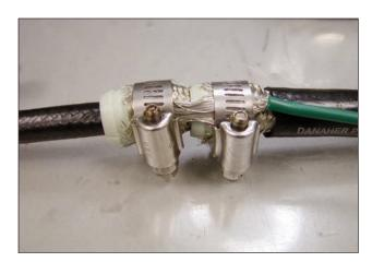
8. Bend the ground conductor back over both couplers and cover both couplers with a 6" heat shrink tubing (PART E). Heat the heat shrink tubing.
