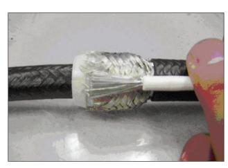
9. Using a conductor clamp (PART C), secure the white neutral conductor to the internal braid layer. Make sure that the clamp is centered on the neutral banding split ring, and tighten with a screwdriver.
