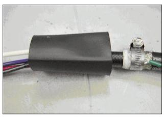
10. Fold the white neutral wire over the clamp and place a 2.5" heat shrink tubing (PART D) over the neutral termination. Heat the heat shrink over the neutral termination.
