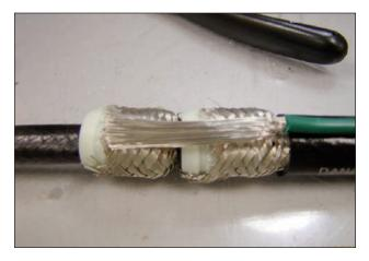
7. Using a conductor clamp (PART C) secure the green ground conductor to the top braid layer.
