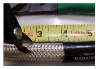
3. Take a ground banding split ring (PART A) and work it underneath the top braid layer. The braid layer should cover as much of the split ring as possible. It may be beneficial to use a tool as shown to open the braid layer making it easier to insert the split ring.
