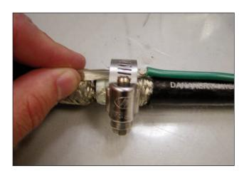
8. Using second conductor clamp (PART C) secure the other side of green ground conductor to the internal braid layer.
